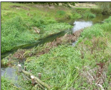
View downstream of the completed woody debris WD 13 and WD14
