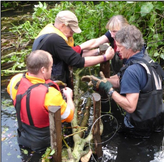
Fixing logs to create WDI
