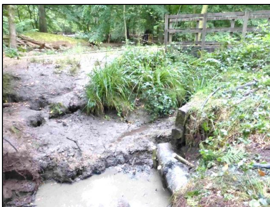
The removed sluice
