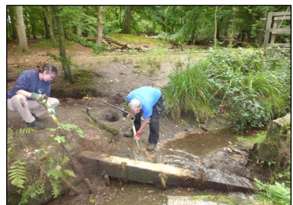
Digging out the sleeper sluice (SL1)
